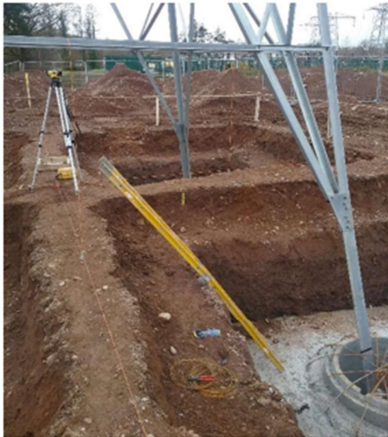
Figure 3-3: Standard 110kV mast foundation excavation. Source: Tli Group
