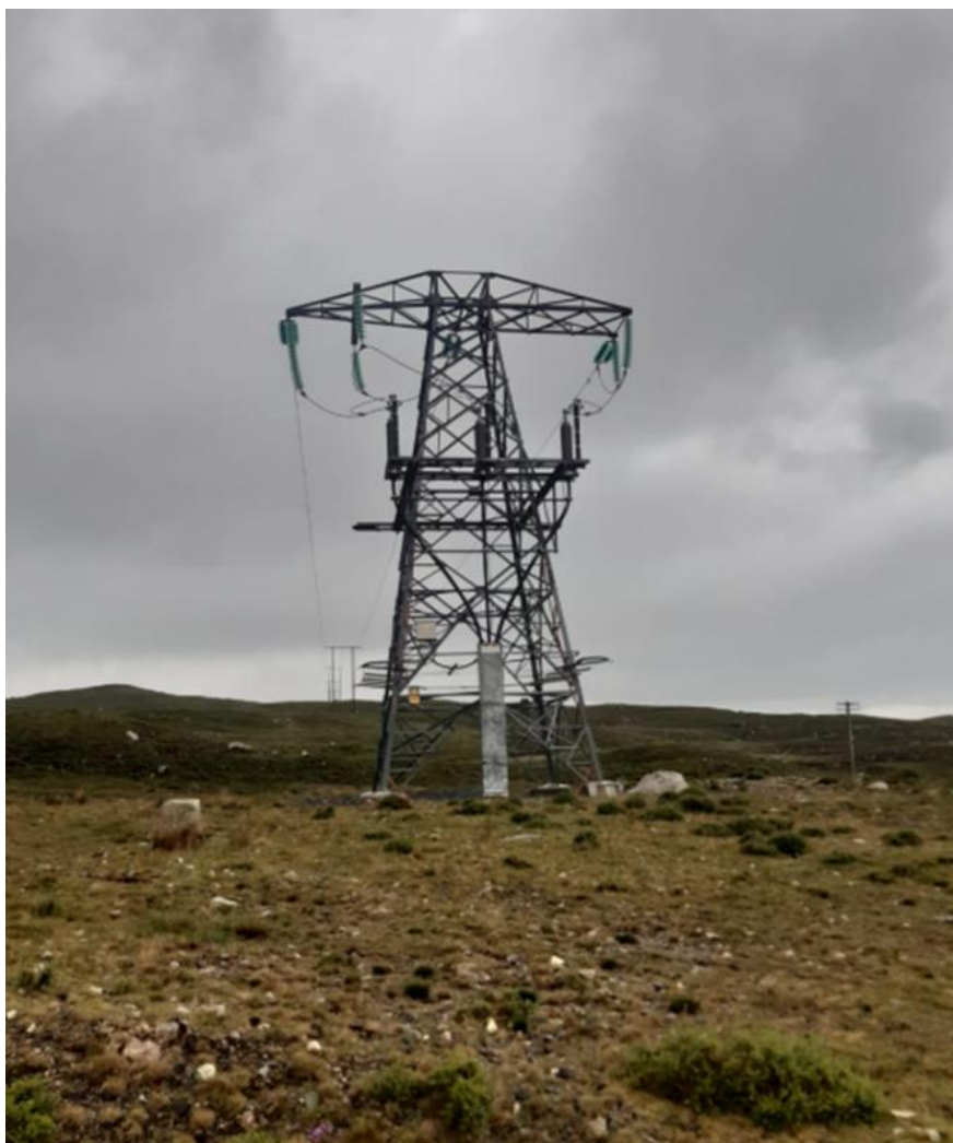
Figure 3-4: Steel Lattice Tower Complete. Source: Applicant, Ardderroo Wind Farm, Co. Galway.
